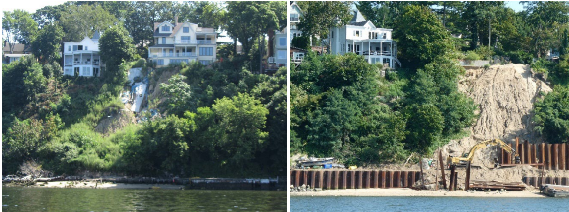
A severe rainstorm in 2017 caused a landslide below Bay Avenue, Sea Cliff (l); the cliff continued to deteriorate, the house was removed, and work is ongoing to shore up the area (photos by Carol DiPaolo, 8/24/17 and 9/12/24)
